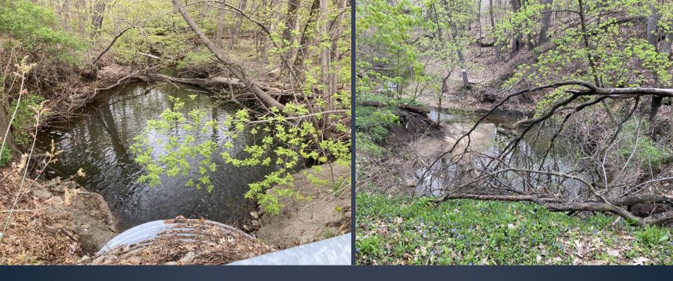
Scour and erosion due to undersized culvert
